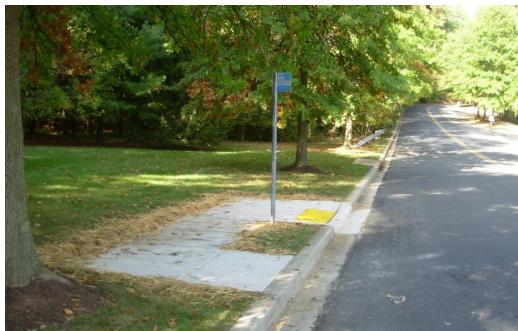
Image of a curb height ADA loading pad for bus stop in Montgomery County, MD
